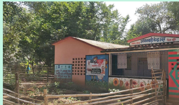
Anganwadi Centre New Building
